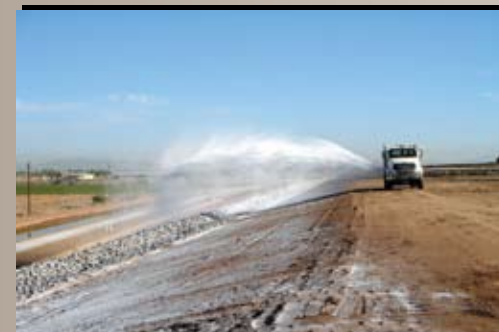
MATERIAL STOCK PILES & SLOPES
