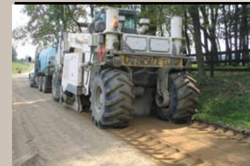
BASE & SUB-BASE SOIL STABILIZATION
