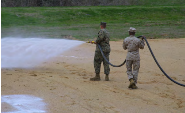
Photo 3. Spraying helipad using hand-held hose
