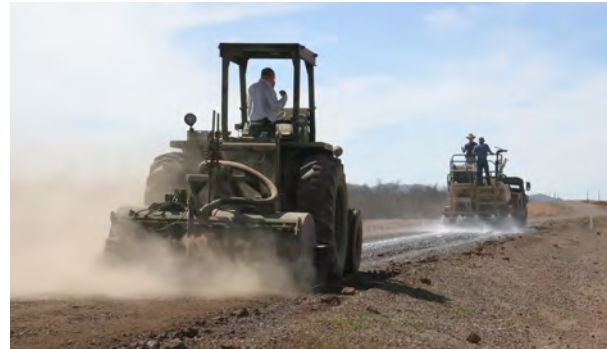
Photo 10. Applying product to road surface and distributing with rotary mixer (steps e,f )
