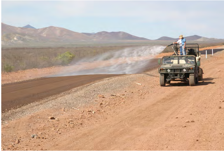
Photo 13. Applying synthetic fluid to road surface using wide-fan nozzle on HydroSeeder
