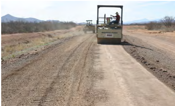
Photo 11. Compacting road surface after tilling (step g )
