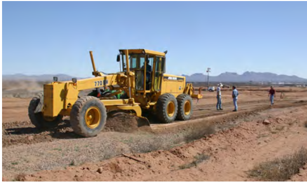
Photo 9. Grading road surface prior to treatment (if needed)
