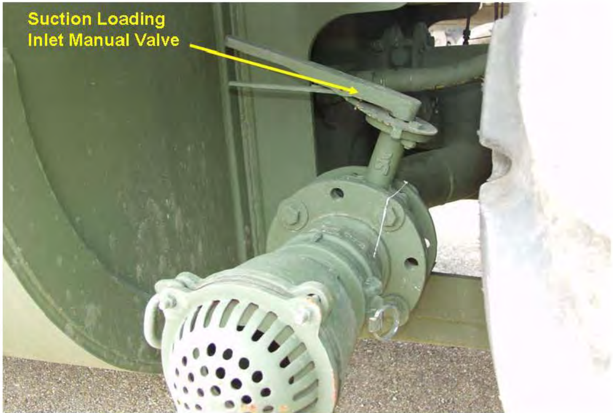
Photo 27. Suction loading inlet manual valve.
