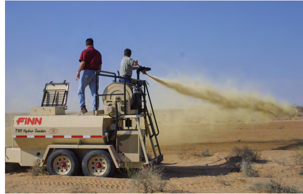
Photo 6. Distributing emulsion onto helipad using tower gun
