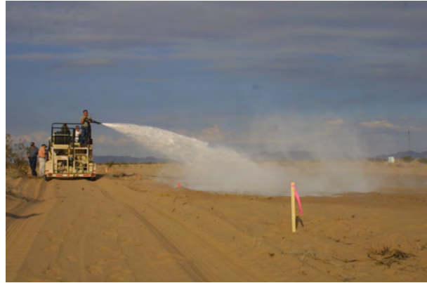
Photo 2. Spraying helipad using tower gun (step d )
