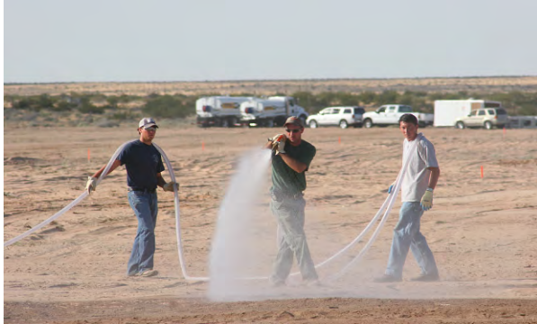
Photo 7. Spraying emulsion with hand-held hose
