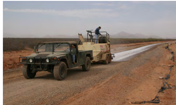
Photo 12. Applying final spray to road surface (step i )
