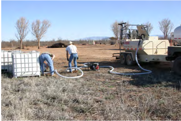
Photo 1. Filling HydroSeeder with product (step b )
